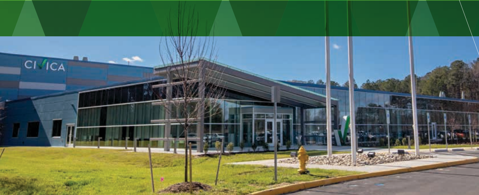
Civica's Petersburg, VA manufacturing facility.
