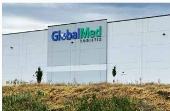
GlobalMed's new distribution center at the Raceway Commerce Center.
