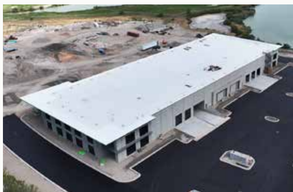
Ratio's facility at Lake Park in West Valley City is nearing completion.
