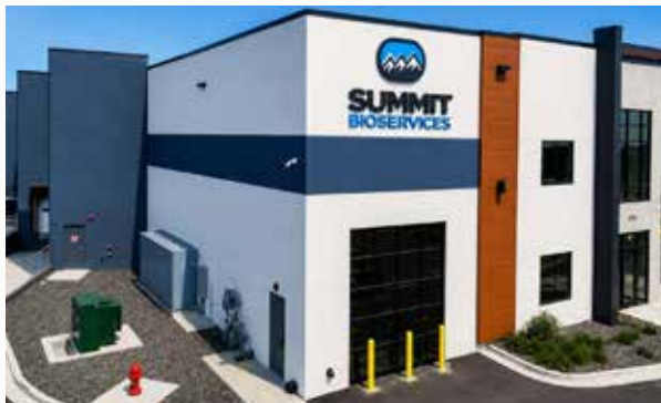
Summit facility at the Lake Park development in West Valley City.
