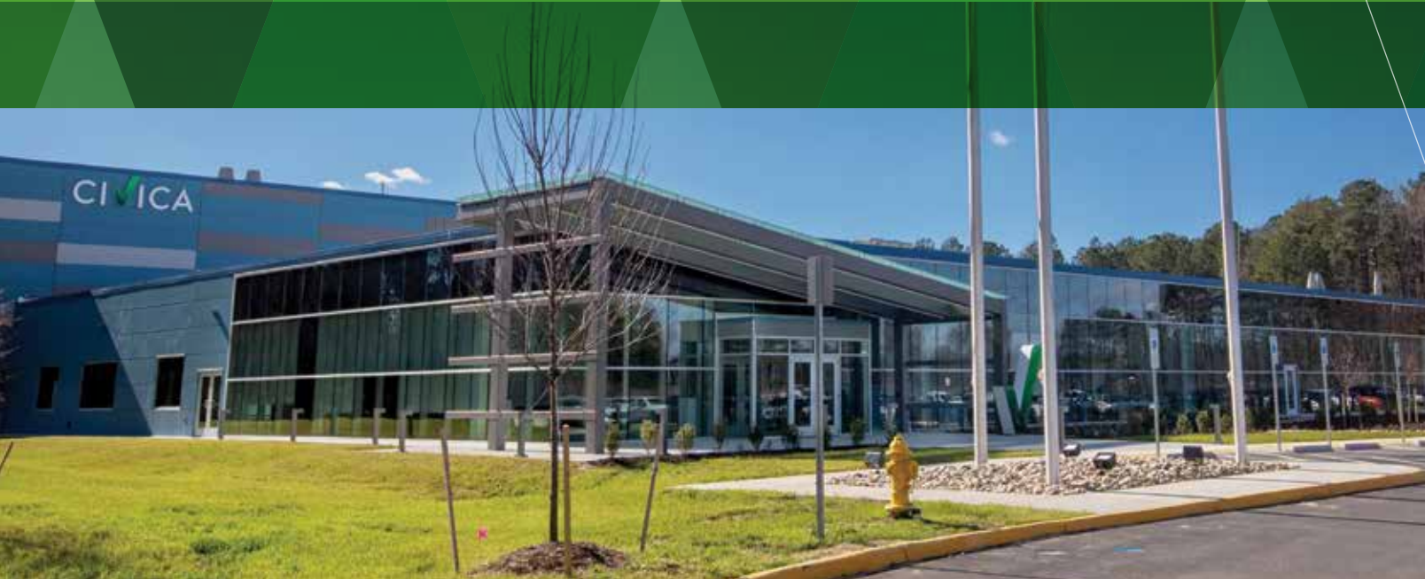
Civica's Petersburg, VA manufacturing facility.
